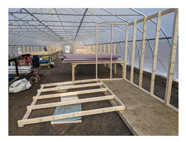
Build the frame of the structure (short sides, long sides, roof, and door frame) using 2x4s. As you can see in the photos, we constructed each side down on the ground and then stood them up to attach.
