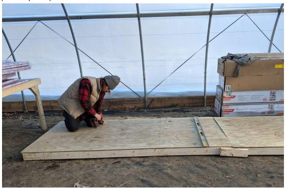
Build bottom frame at dimensions of 4'x16', with at least 5 interior cross pieces.
