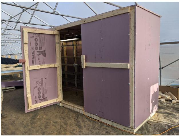
Construct a door out of 2x4s and foam board Mount with hinges Secure with a makeshift wooden spin latch
